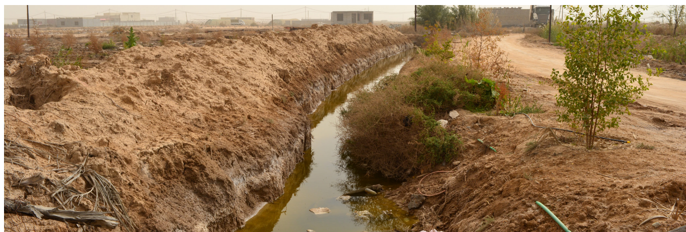
Picture 2: Contaminated stagnant water in irrigation canals
